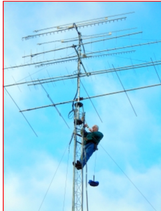
Ed, WA3BZT putting the finishing touches On the 7/8" hardlines for 2304 & 34356
